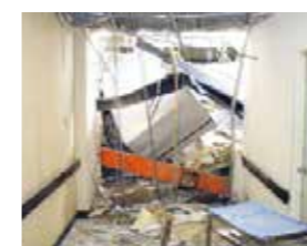
Collapsed corridor in a hospital after the disaster (source: Hoshi General Hospital Foundation)
